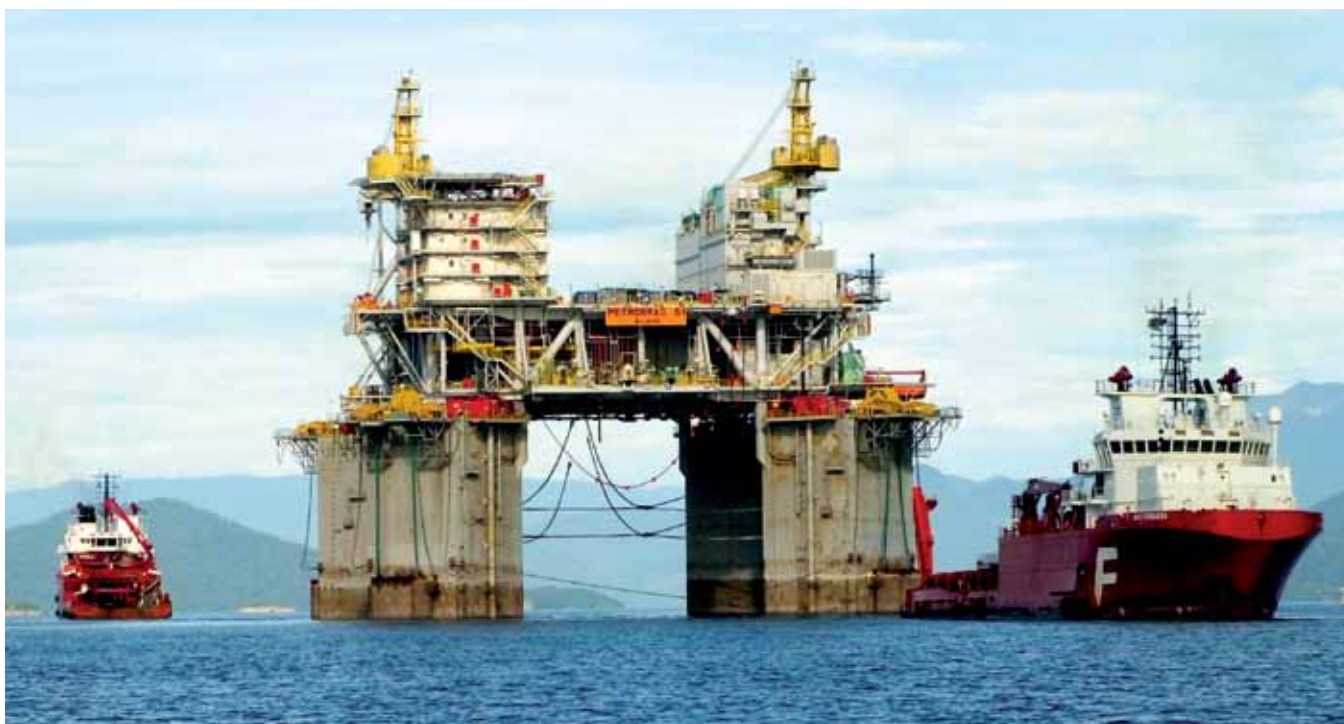
Designed by FloaTEC LLC, a joint venture between Keppel FELS and McDermott, P-61 is the first TLWP to be built in Brazil
